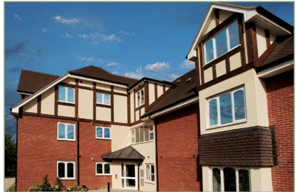
Riverdale House, Endenbridge, Kent
